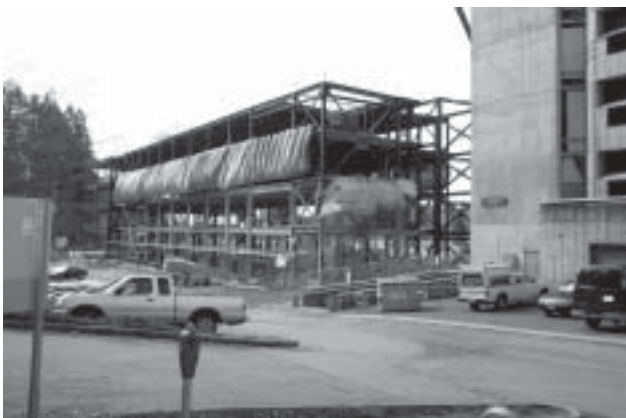
Communications Facility - Northeast Elevation
