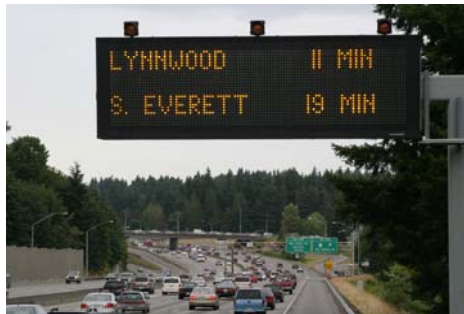
Photo 9: Variable message sign on I-5 provides driver information such as travel times and warnings of incidents ahead.
