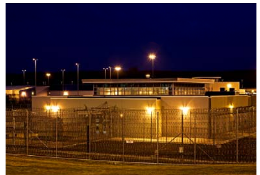
Photo 3: Stafford Creek Correctional Center replaced all perimeter lighting, resulting in an estimated power savings of 27 percent over the old system.
