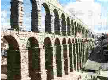
Segovia's Roman Aqueduct
