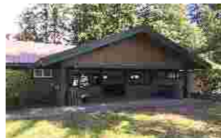
Upper Picnic Shelter
